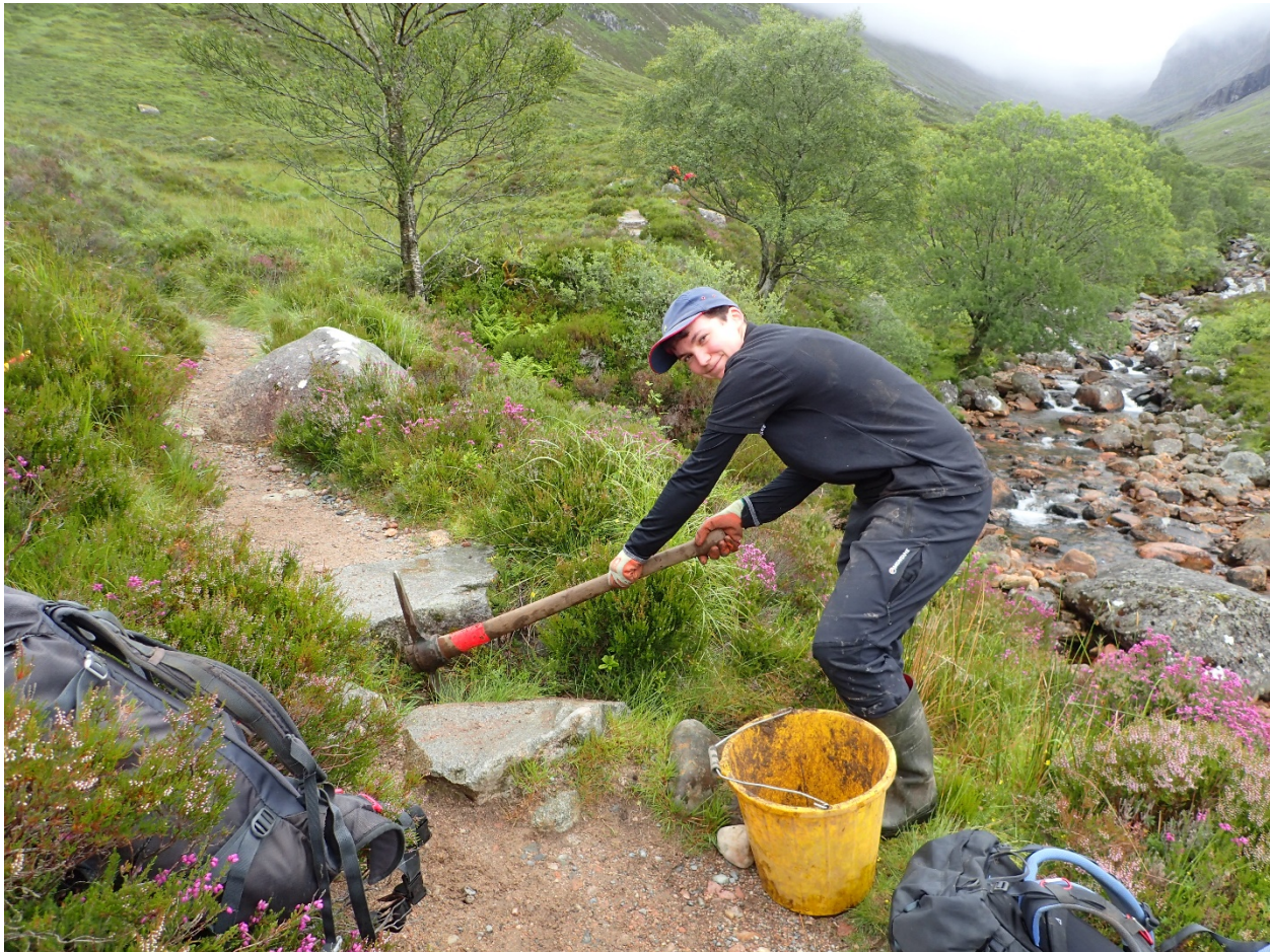
Figure 15: Ellie clearing the cross drains on the Allt a’Mhuilinn
