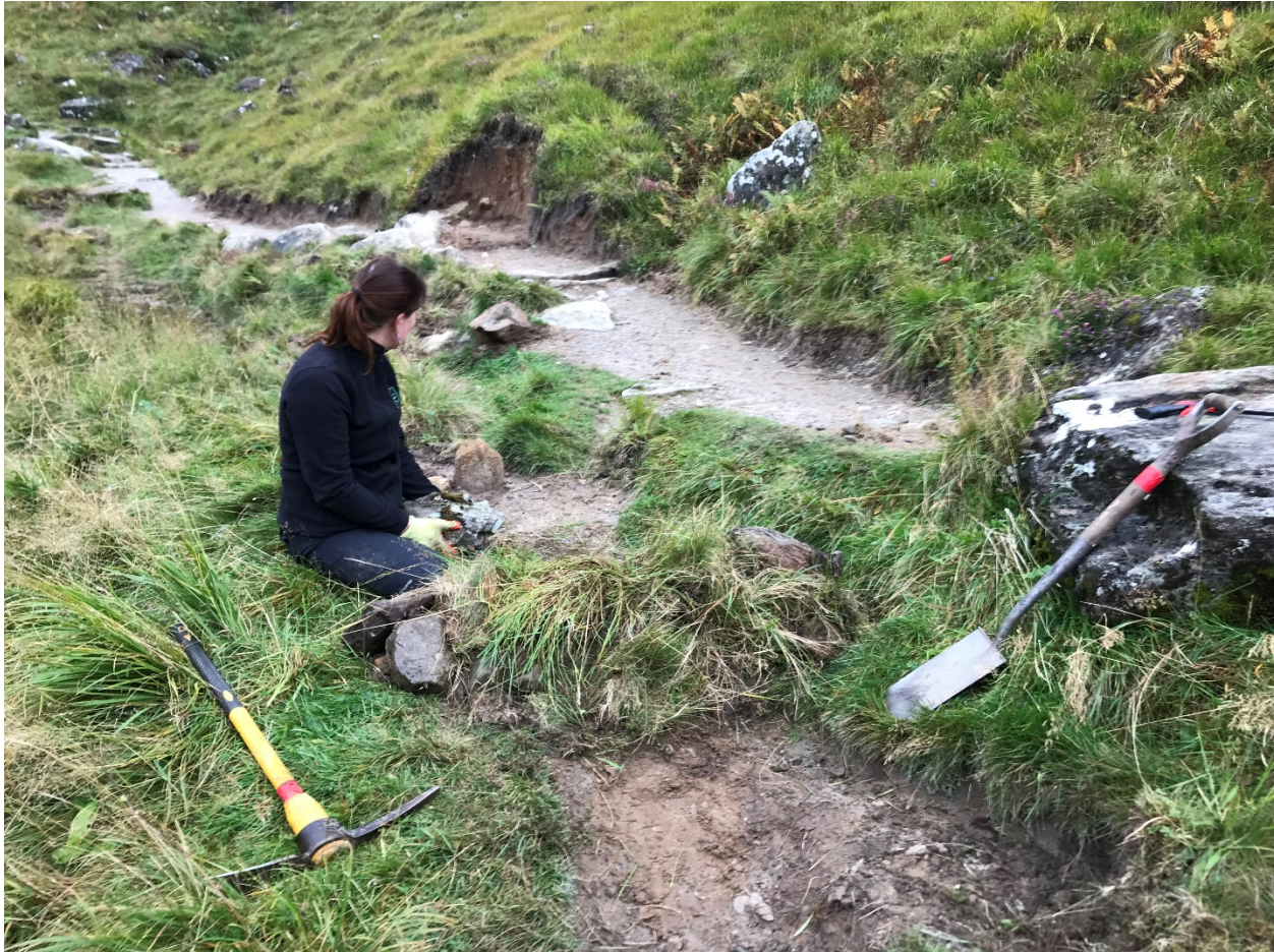
Figure 20: Charlotte reducing the impacts of braiding on the Steall Meadows path
