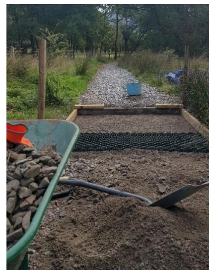
Figure 14. All Abilities Path repairs (Rangers, 2021)
