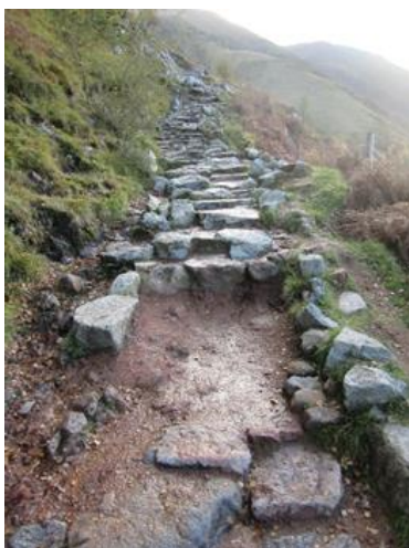
Figure 19. Mountain path to stop collapsing stone (Rangers, 2021)
