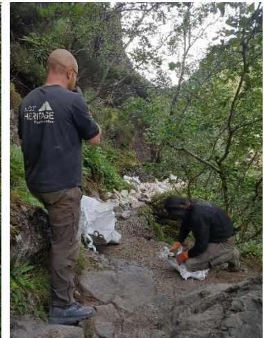
Figure 11. Contractors working on path repairs (Rangers, 2021)
