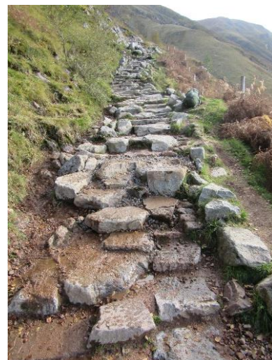
Figure 20. After completion (Rangers, 2021)
