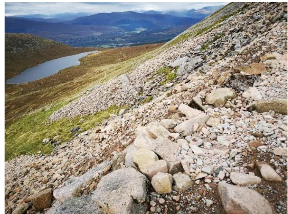
Figure 9. Finished revetment (After) (Rangers, 2021)
